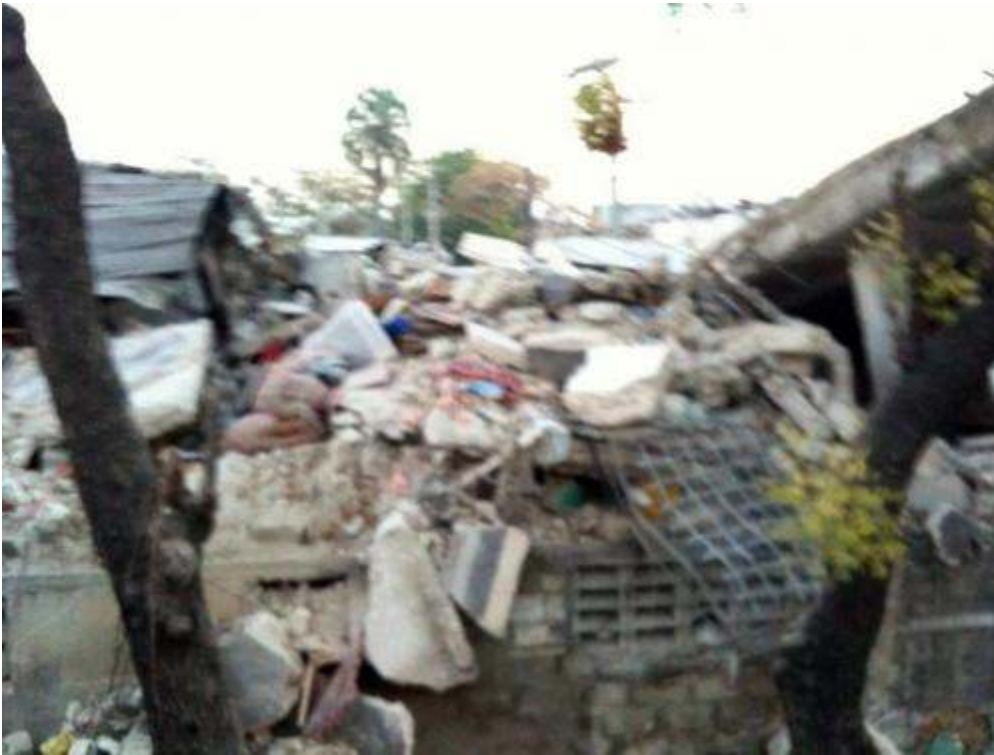
Destroyed building next to our clinic
